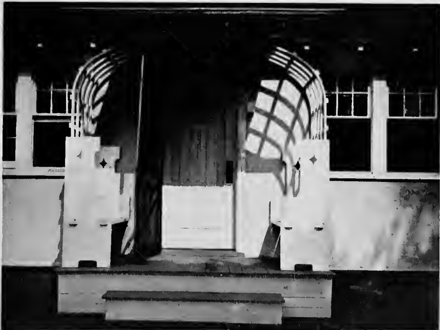
The entrance porch is not large, merely a small platform with seats sheltered by a vine lattice
